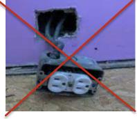
Outlets outside are required to have a cover, and be GFCI protected when near a water source/wet location.
