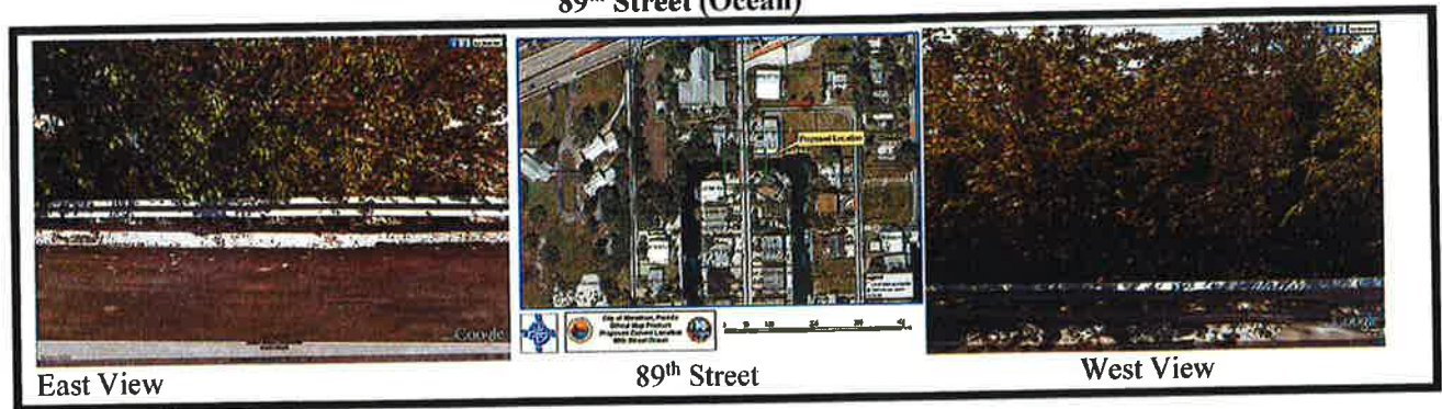
Figure 4. 89 th Street (Ocean) Street and Areal Views.
