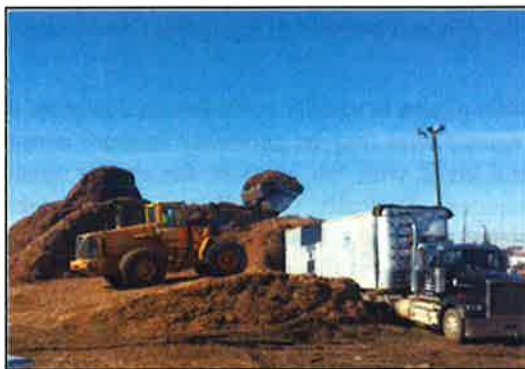
Mulch Haul Out for Beneficial Re-use – Augusta, GA
