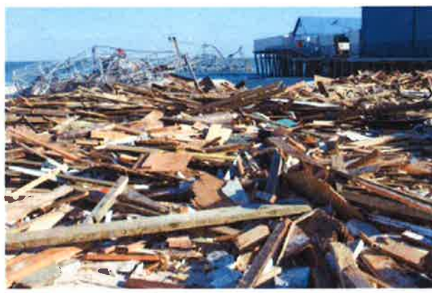
Figure 1: Hurricane Sandy Debris along the Historic Boardwalk in Seaside Heights, New Jersey. Source: FEMA
